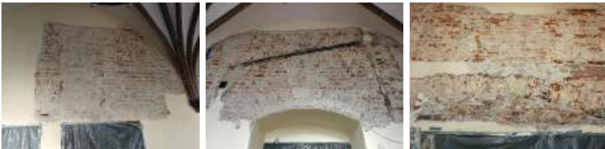
Fig. 167. Invasive research conducted in the sacristy of St. Nicholas Church, 2019, showing plaster removal. Source: author.
