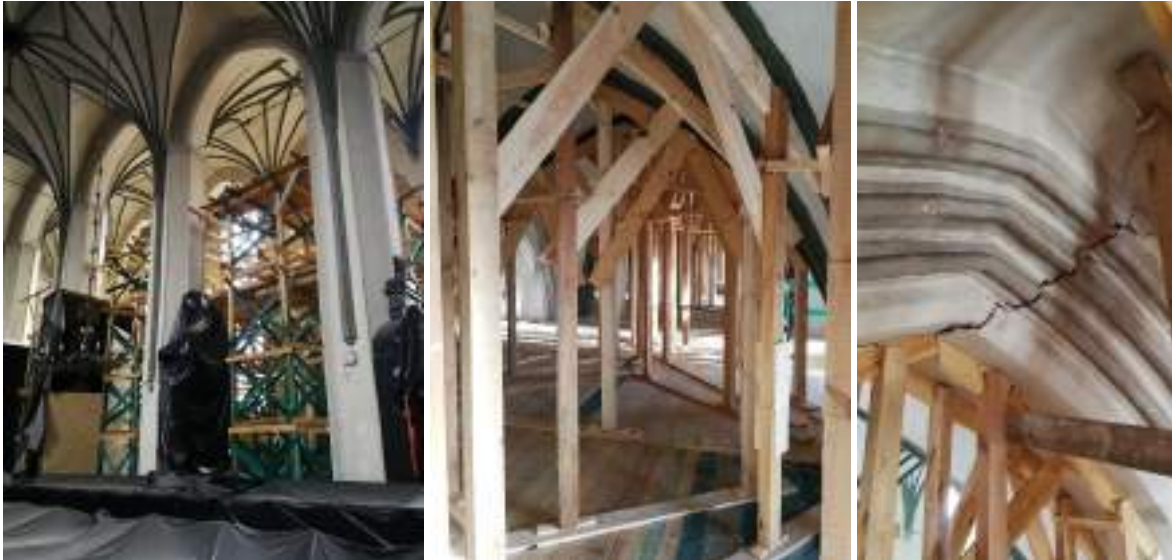
Fig. 166. Support structure in the southern nave with vertical shoring and visible crack in the arcade. Source: author.
