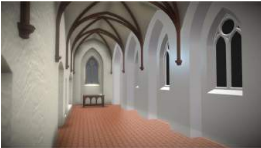
Fig. 177. Original design of a simple five-span cross-ribbed vault sacristy, ca. 1348. The southern wall is shown in transparent form to indicate the hypothetical layout 845 . Source: author and Piotr Samól.
