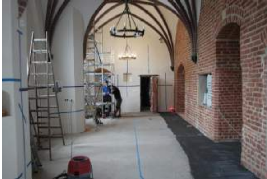
Fig. 170. Sacristy during conservation works, with blue markers introduced for photogrammetry scanning. Source: author.
