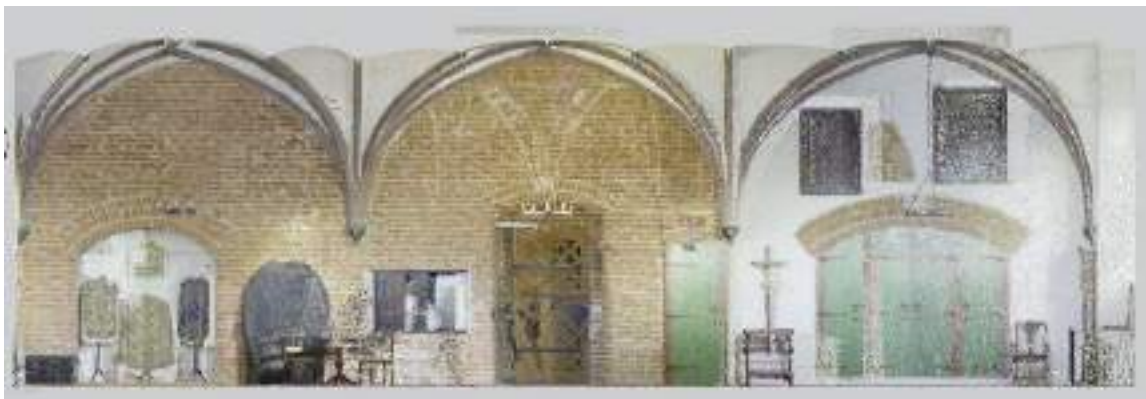
Fig. 173. Cross-section of the sacristy represented as a laser point cloud after conservation works, showing the northern wall with visible masonry anomalies that confirm the existence of earlier vaulting systems. Registered in February 2023. Source: author
