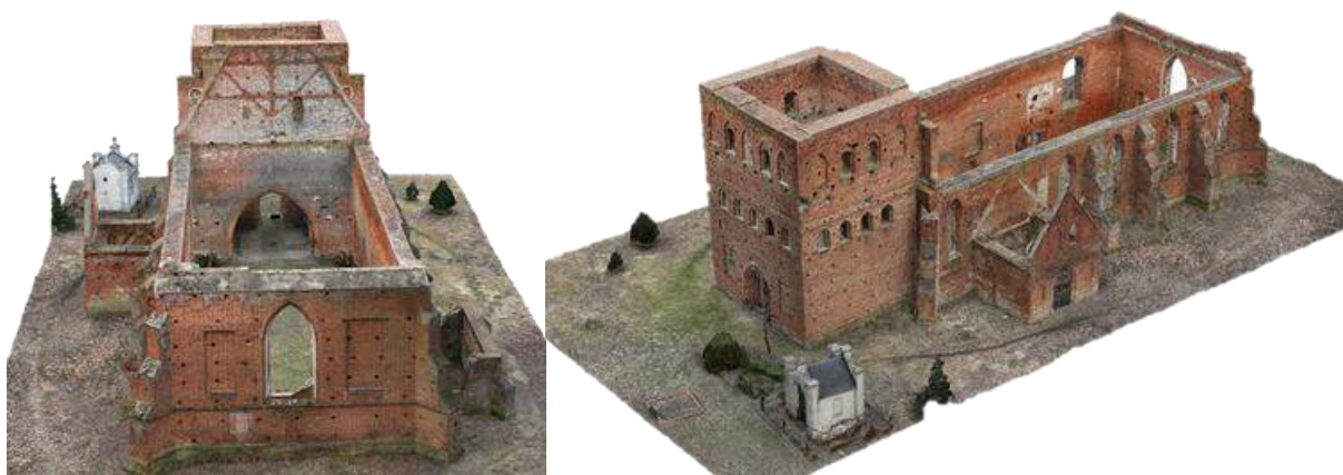
Fig. 144. Architectural scale photogrammetry: textured 3D mesh model of the church ruins in Steblewo. Source: author 787 .
